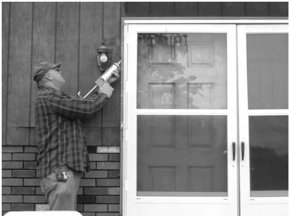
AEOA Weatherization staff caulking a residential door.
